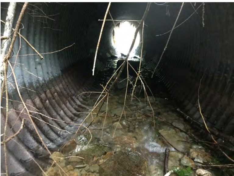
Looking through culvert from inlet
